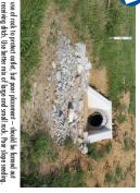
Fair use of rack to protect outlet, but poor placement – should be fanned out into receiving ditch. Use better mix of large and small rack. Poor slope seeding
