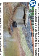
Good construction and operation. Note long basin design, seeded sidewalls, and flow restrictor (half-jape and rock berm) in front of inlet hole.
