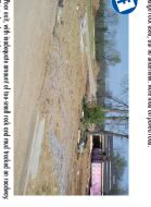
Poor exit, with inadequate amount of too-small rock and mud tracked on roadway. This is clearly a violation.
